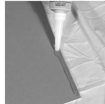
4 - Run E-6000 along outer edge of the top of mat.
